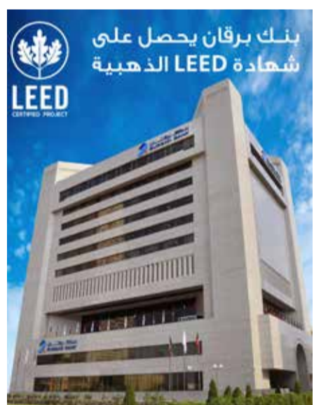
Burgan Bank achieves LEED Gold certification for Operations and Maintenance.
