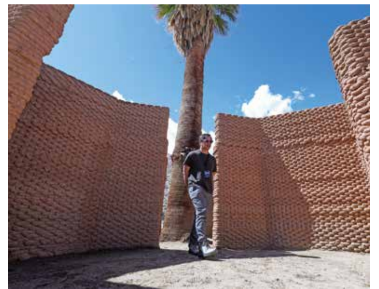
A visitor walks through Ronald Rael's piece "Adobe Oasis," which used a robotic arm to 3D print walls made of clay and straw, in the traditional local adobe.
