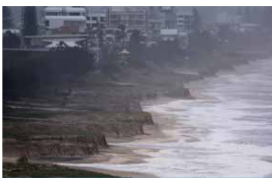
GOLD COAST: A general view shows erosion at Miami Beach after the sand was washed away during Tropical Cyclone Alfred on the Gold Coast on March 9, 2025. — AFP
