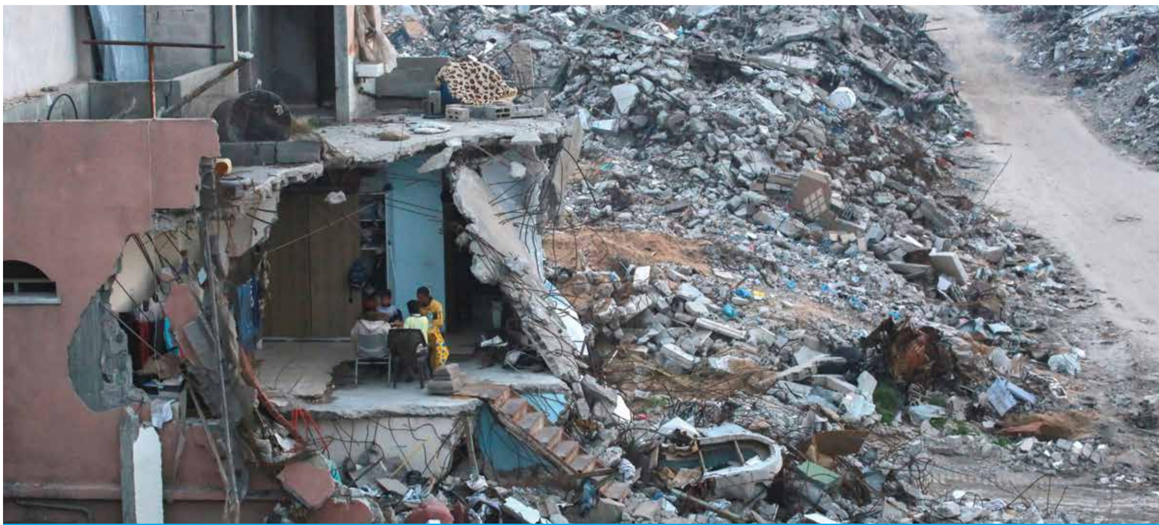
BEIT LAHIA: A Palestinian family eat an iftar meal in their destroyed house amid the rubble of buildings in Beit Lahia in the northern Gaza Strip on March 4, 2025. — AFP
