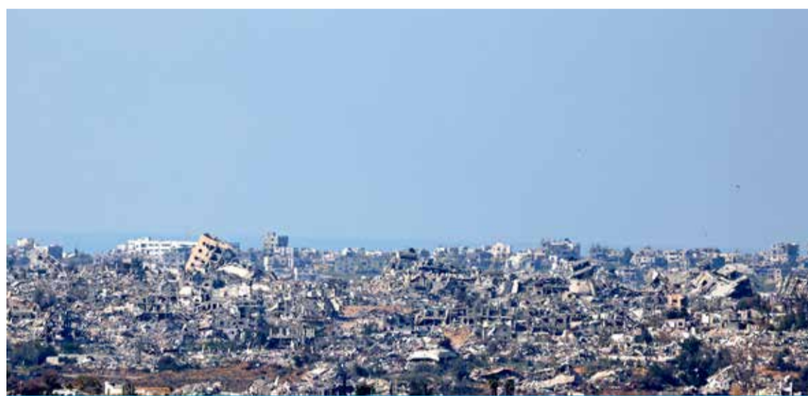
This picture shows the damaged and destroyed buildings in the northern Gaza Strip, on January 19, 2025.
