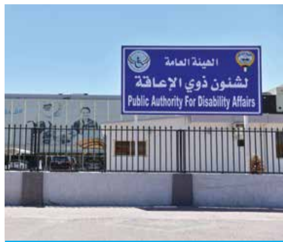
KUWAIT: The Public Authority for Disability Affairs building is seen in this photo. — KUNA
