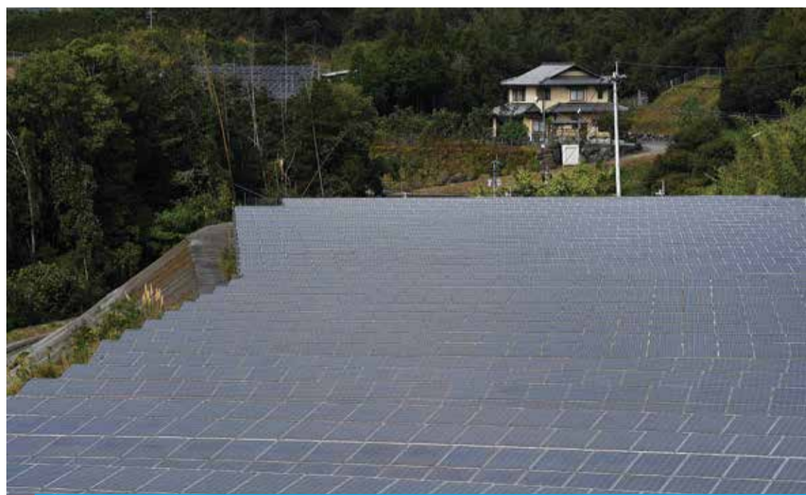
YUFU: Solar panels are pictured in Yufu, Oita prefecture. Japan wants renewables to be its top power source by 2040, as it pushes to become carbon neutral by mid-century, according to draft government plans unveiled on December 17, 2024. — AFP
