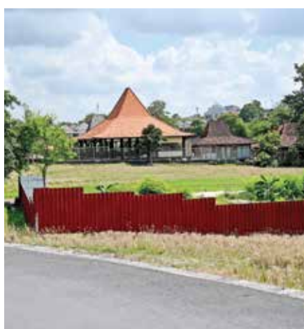
This photo shows a villa under construction next to rice fields in Canggu, Badung regency on Bali island.
