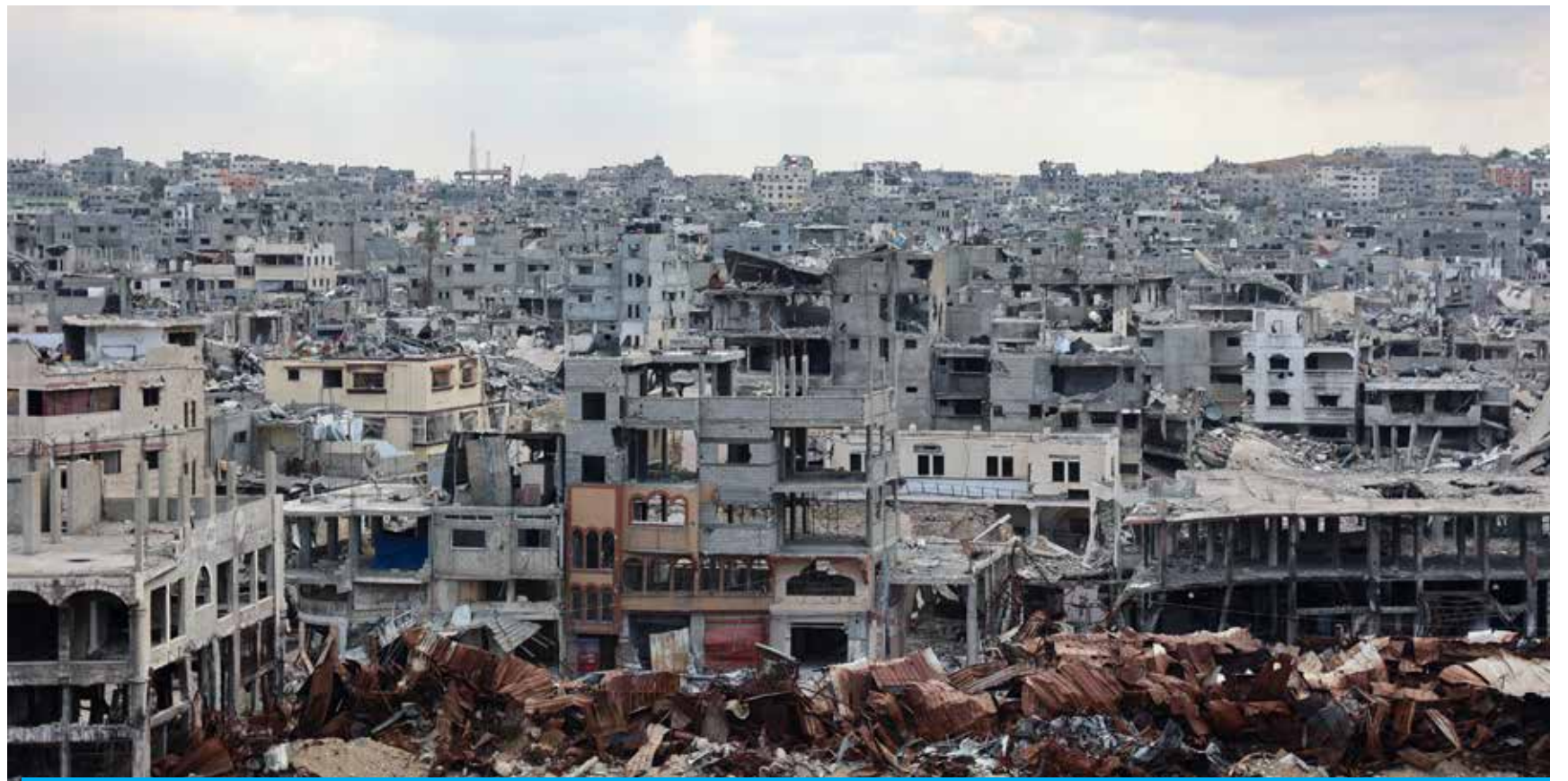
GAZA CITY: Buildings are destroyed in the Shujaiya neighborhood of Gaza City on October 7, 2024, on the first anniversary of the Zionist military offensive in Gaza. — AFP
