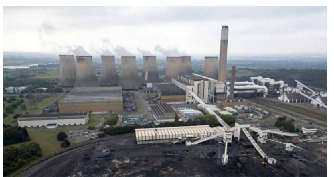
An aerial view of the Ratcliffe-on-Soar coal-fired power station near Nottingham in central England, seen on Sept 19, 2024. — AFP
