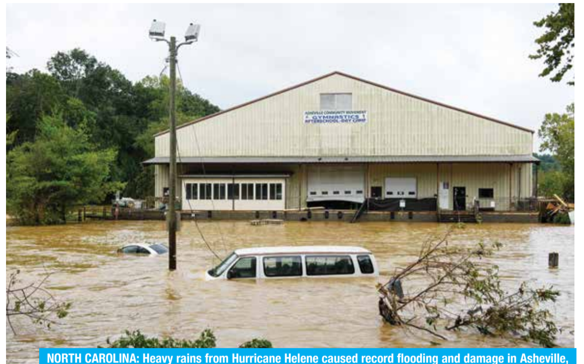
NORTH CAROLINA: Heavy rains from Hurricane Helene caused record flooding and damage in Asheville, North Carolina. — AFP
