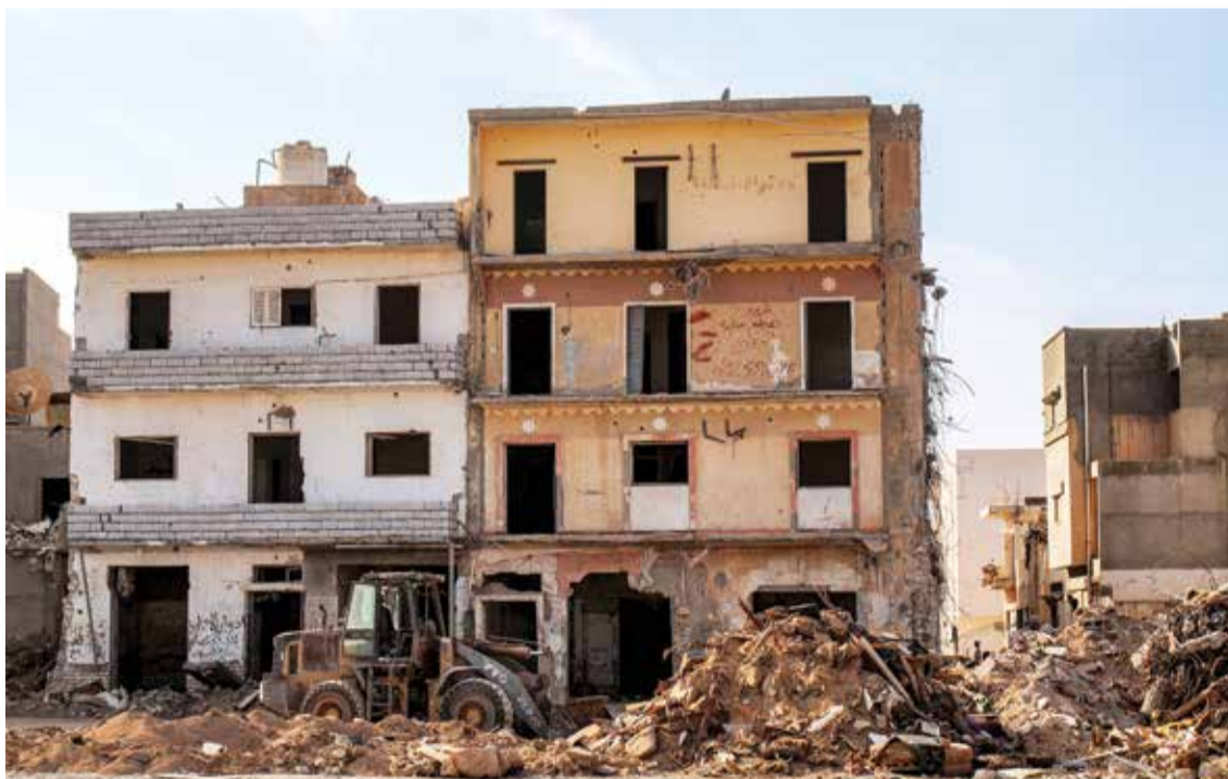
DERNA: A bulldozer moves past damaged buildings during ongoing reconstruction work in Libya's eastern coastal city of Derna on September 9, 2024. — AFP
