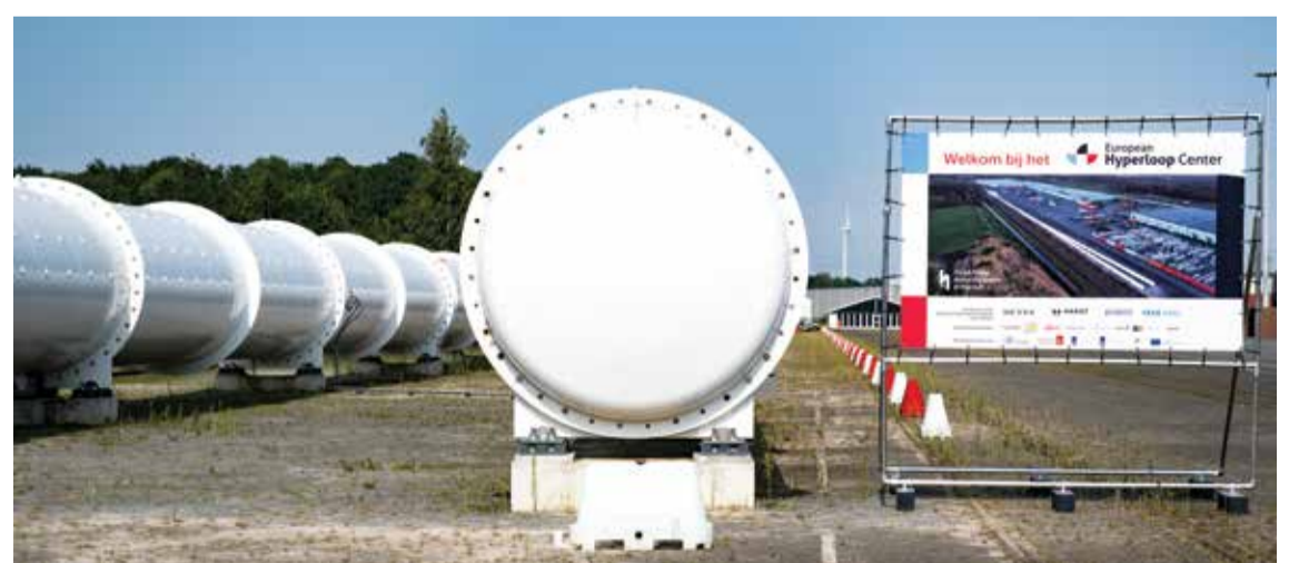
VEENDAM, Netherlands: A view shows the end of a Y-shaped 420-metre (1,377-foot) white tunnel at the European Hyperloop Center (EHC) in Veendam, on Sept 7, 2024. — AFP
