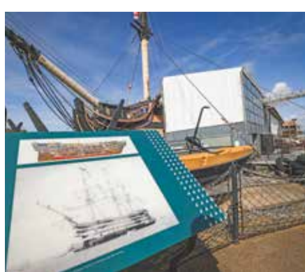
A temporary structure shrouds HMS Victory.
