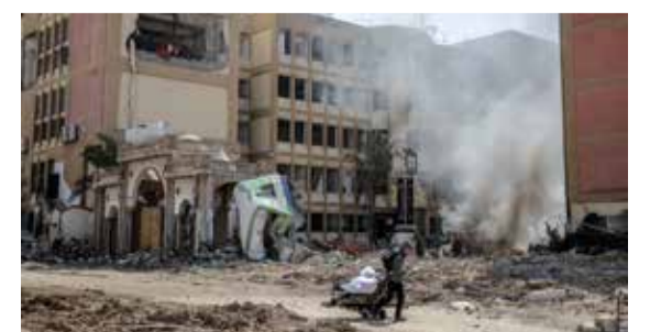
GAZA: A young Palestinian pulls a wheel cart past the heavily damaged building of Al-Azhar University in this file photo. — AFP
