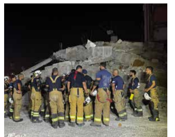
KUWAIT: Rescuers work at a collapsed building in Jabriya on Aug 21, 2024. — KUNA
