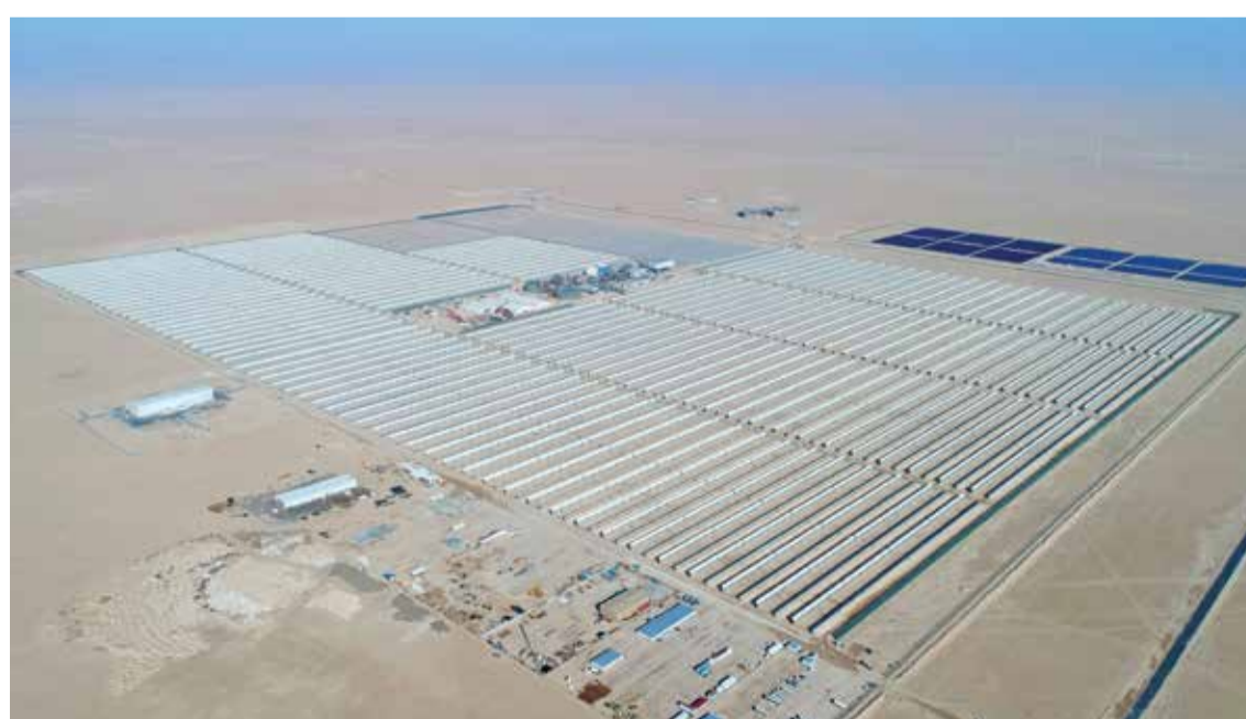
JAHRA: Part of the Al-Shagaya Concentrated Solar Power Project is seen in this photo taken from the Kuwait Institute for Scientific Research website.
