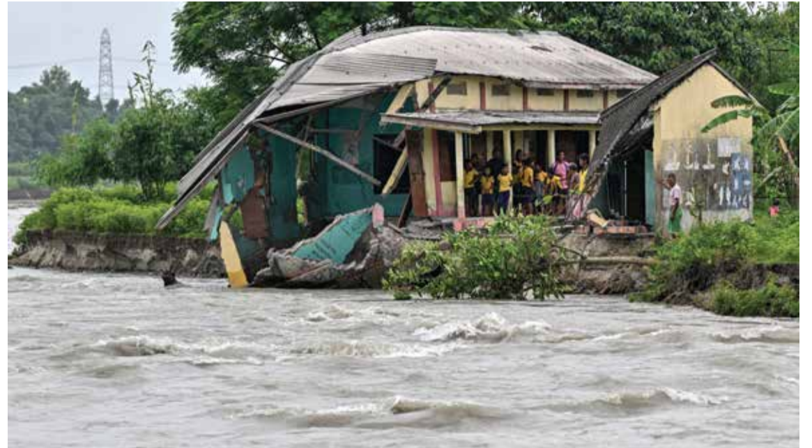
KOKRAJHAR: Students and villagers stand outside a partially collapsed government school following severe soil erosion after an increase in the water level of the Sermanga river during monsoon season in the New Bongaigaon village of Kokrajhar district in India's Assam state on August 10, 2024. — AFP
