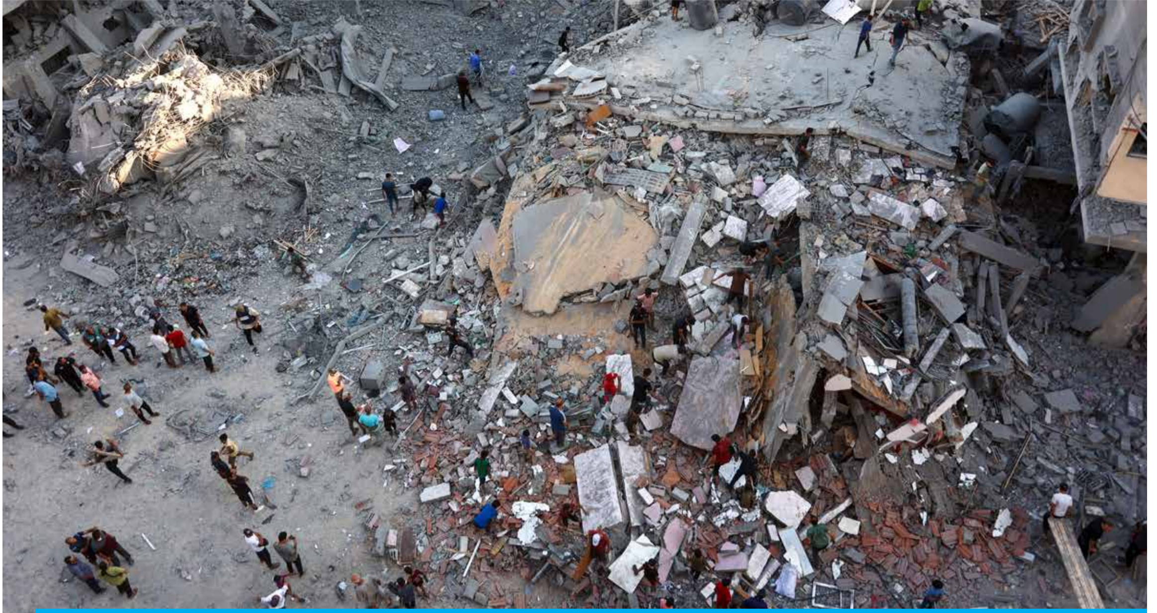
GAZA: People inspect the damage in Gaza City's Sheikh Radwan neighborhood following Zionist bombardment on August 11, 2024. — AFP
