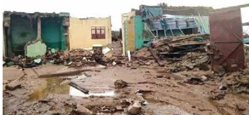
Photos show ruined infrastructure due to the recent floods in Yemen. — KUNA photos
