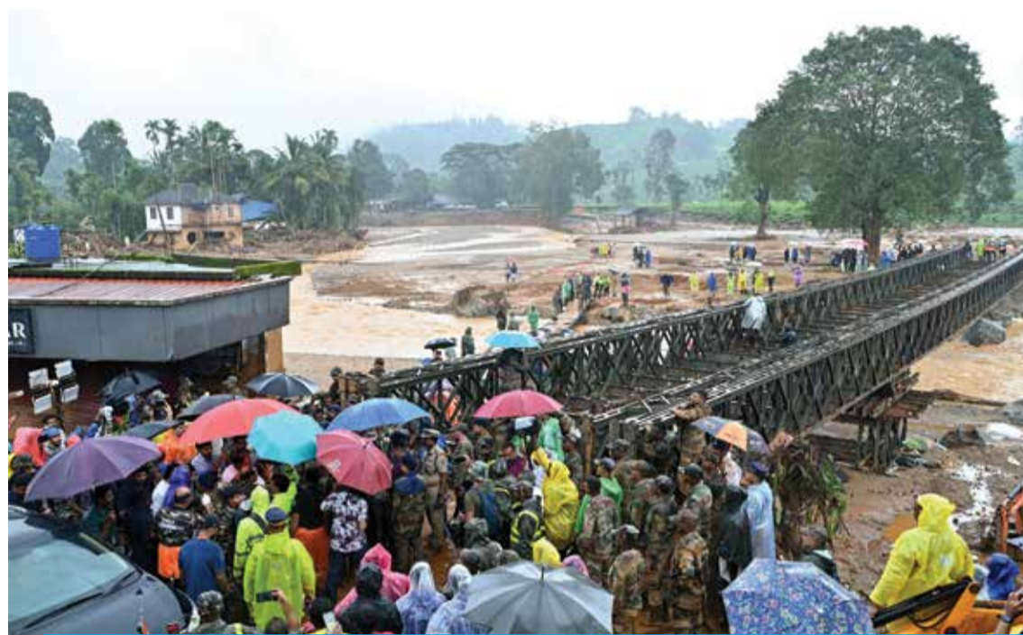
WAYANAD, India: A makeshift bridge has been installed for the rescue operation after the landslides in Wayanad on August 1, 2024. — AFP
