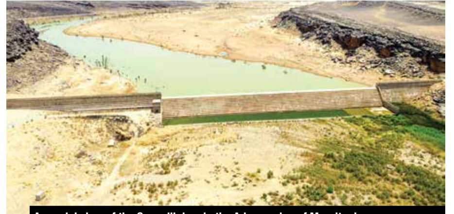
An aerial view of the Seguelil dam in the Adrar region of Mauritania.
