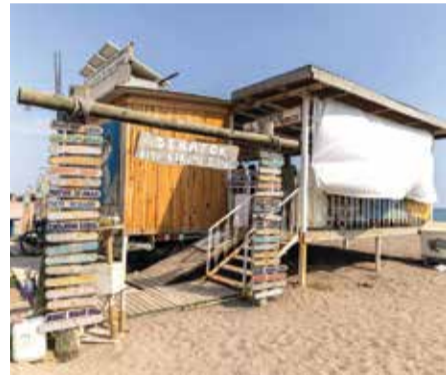
The Dekafok information and observation centre in Manavgat.
