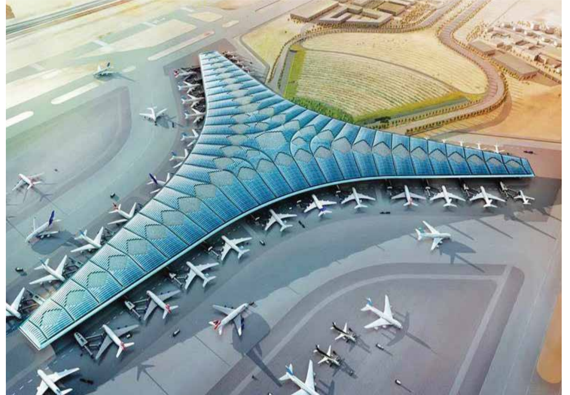
The new airport passenger terminal project (T2).
