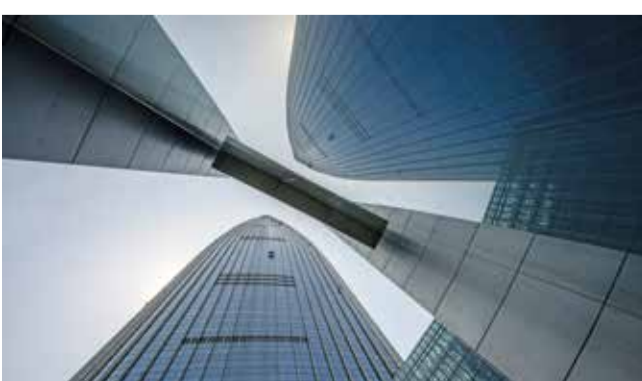
This photo shows a special "gondola" (top center) used by window cleaners high up on the Lotte World Tower, South Korea's tallest building, in Seoul.
