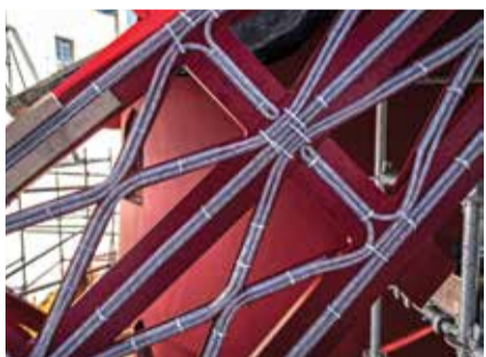
A detail view shows the neon tubes on one of the four temporary windmill sails installed on the top of the Moulin Rouge cabaret following the collapse of the former ones, in Paris.
