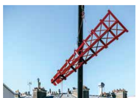
This photograph shows a crane lifting one of the four temporary windmill sails during its installation on top of the Moulin Rouge cabaret following the collapse of the former ones, in Paris.
