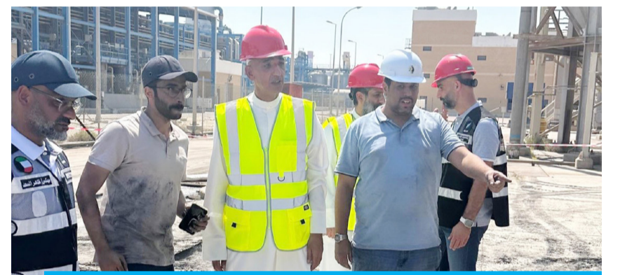
KUWAIT: Minister of Electricity and Water and Renewable Energy Mahmoud Bushehri visits the Al-Zour South power plant after a fire broke out in a unit on June 23, 2024.
