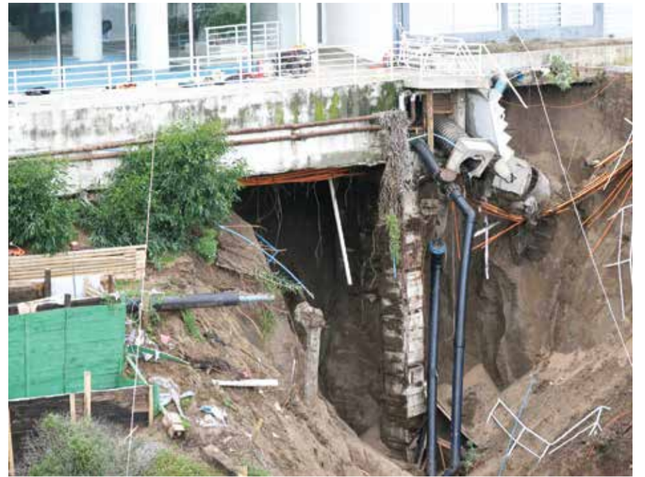
View of a building that suffered a sinkhole in its structure due to rainwater accumulation.
