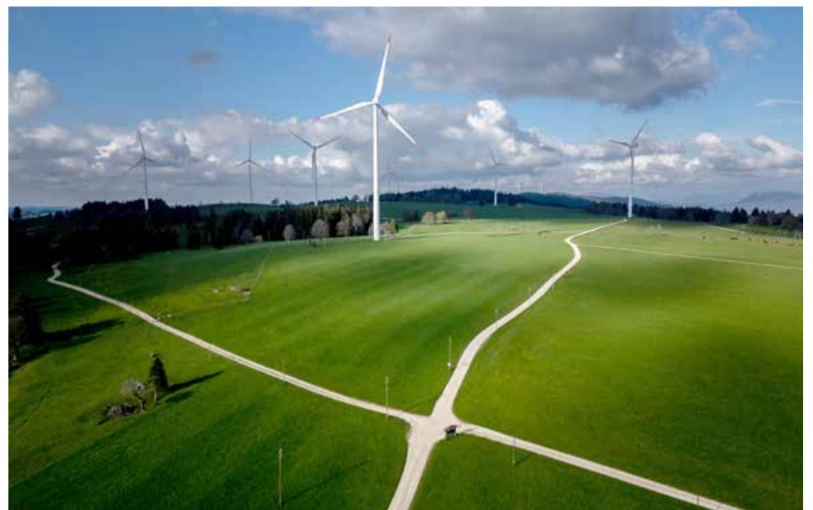
SAINT-IMIER, Switzerland: This photograph taken on May 8, 2024 shows wind turbines in Mont Soleil mountain, above Saint-Imier, ahead of a nationwide vote on a new electricity law. — AFP
