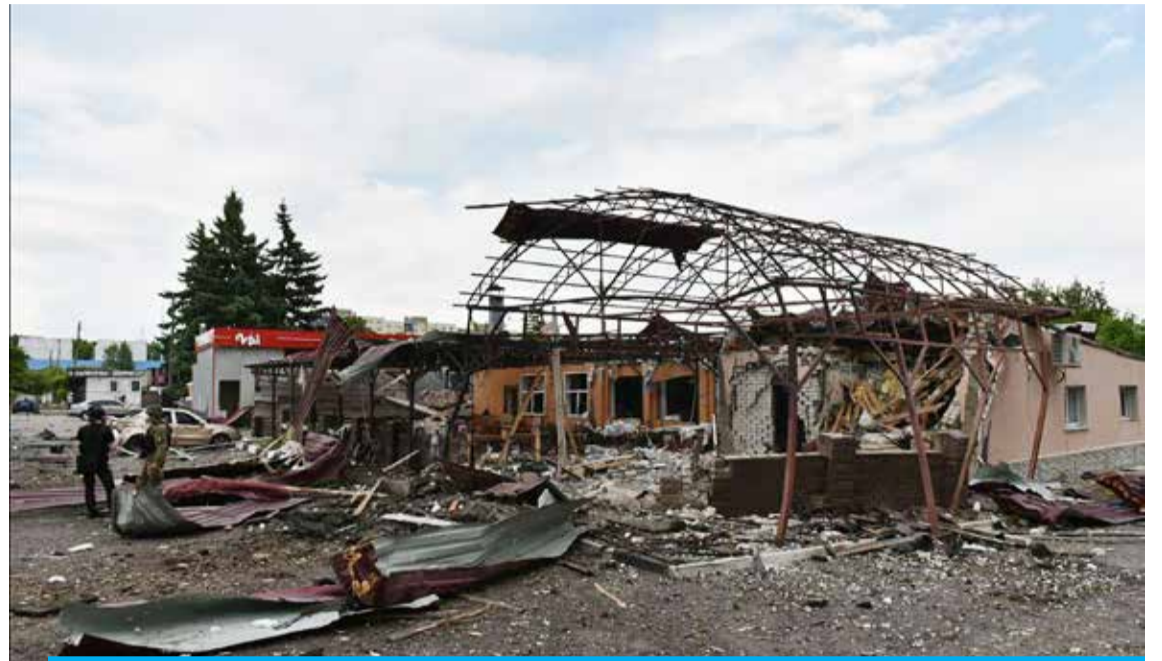
KHARKIV: This handout photograph shows buildings destroyed as a result of a shelling in Kharkiv, amid the Russian invasion of Ukraine. — AFP
