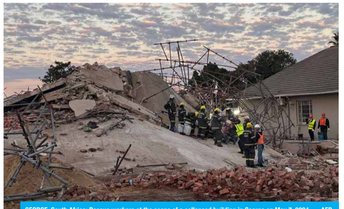
GEORGE, South Africa: Rescue workers at the scene of a collapsed building in George on May 7, 2024. — AFP
