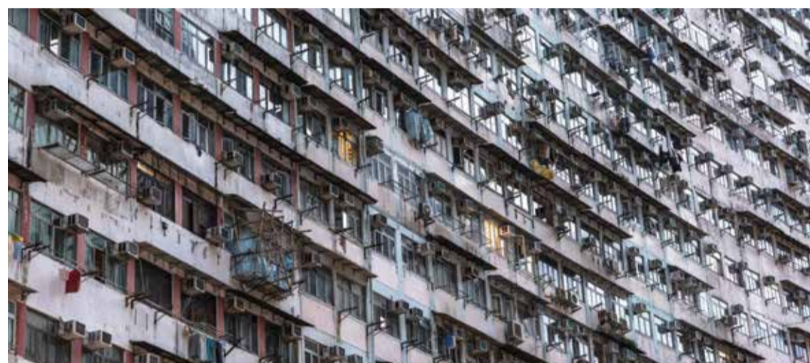
This picture taken on April 29, 2024 shows air conditioning units on an apartment building in Hong Kong. — AFP
