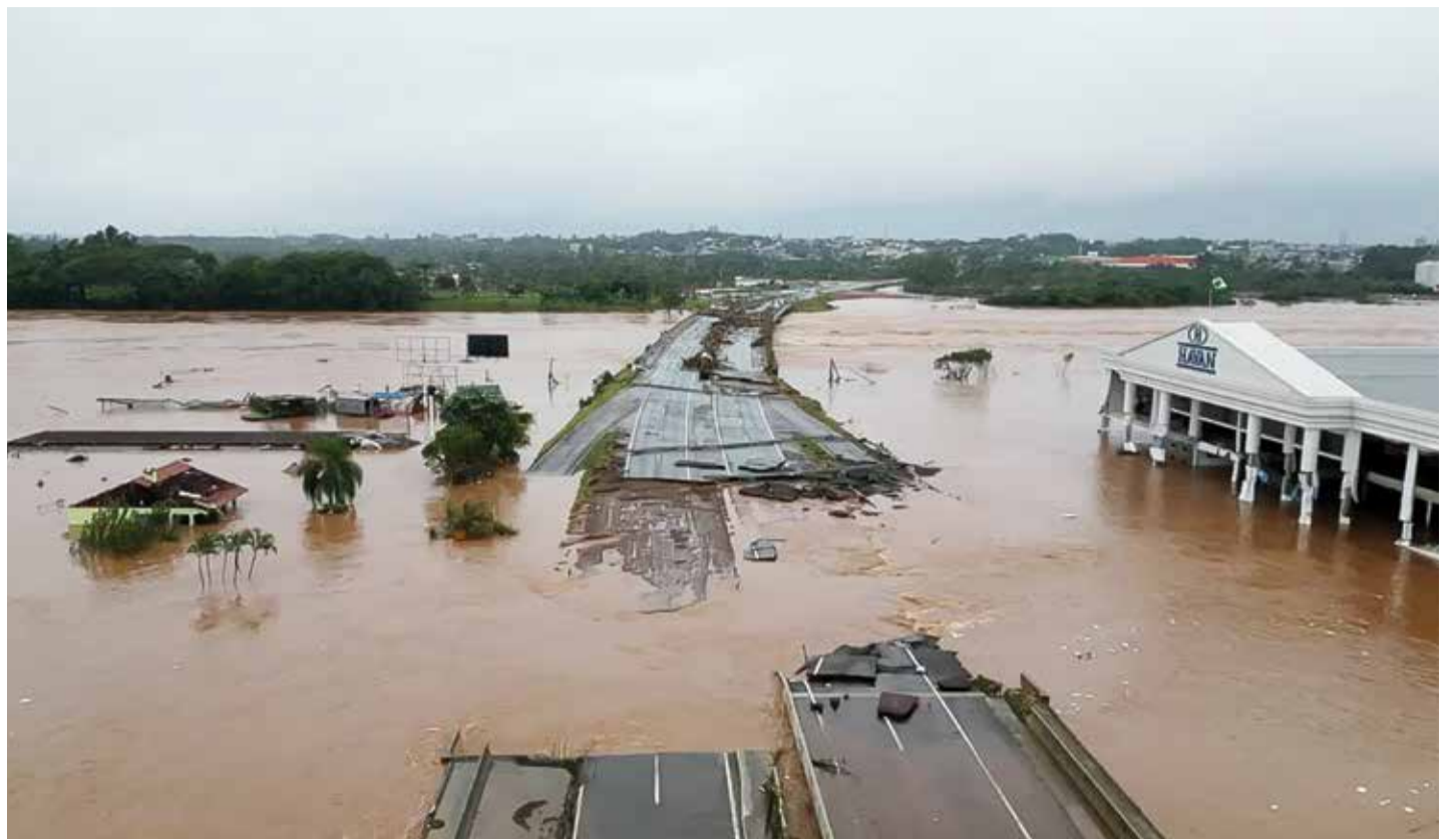
Grab from a handout video released by the Sao Paulo Civil Defense showing the flooded Taquari river bridge, which is part of the BR-396 highway that connects the cities of Lageado and Estrela, in the region of Vale do Taquari, Rio Grande do Sul state, Brazil on
