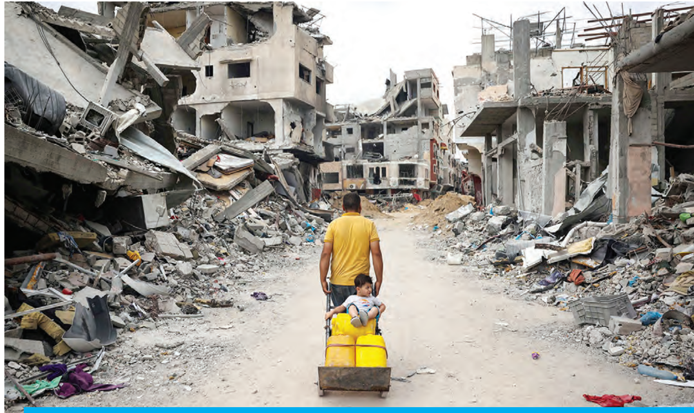
GAZA: A Palestinian man pulls a cart on a road lined with destroyed buildings in Khan Yunis in the southern Gaza Strip on May 2, 2024. — AFP
