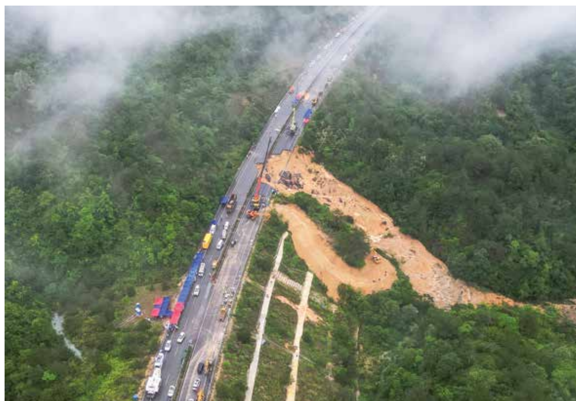
MEIZHOU, China: This photo taken on May 1, 2024 shows an aerial view of a collapsed section of a highway near Meizhou, in southern China's Guangdong province. - AFP
