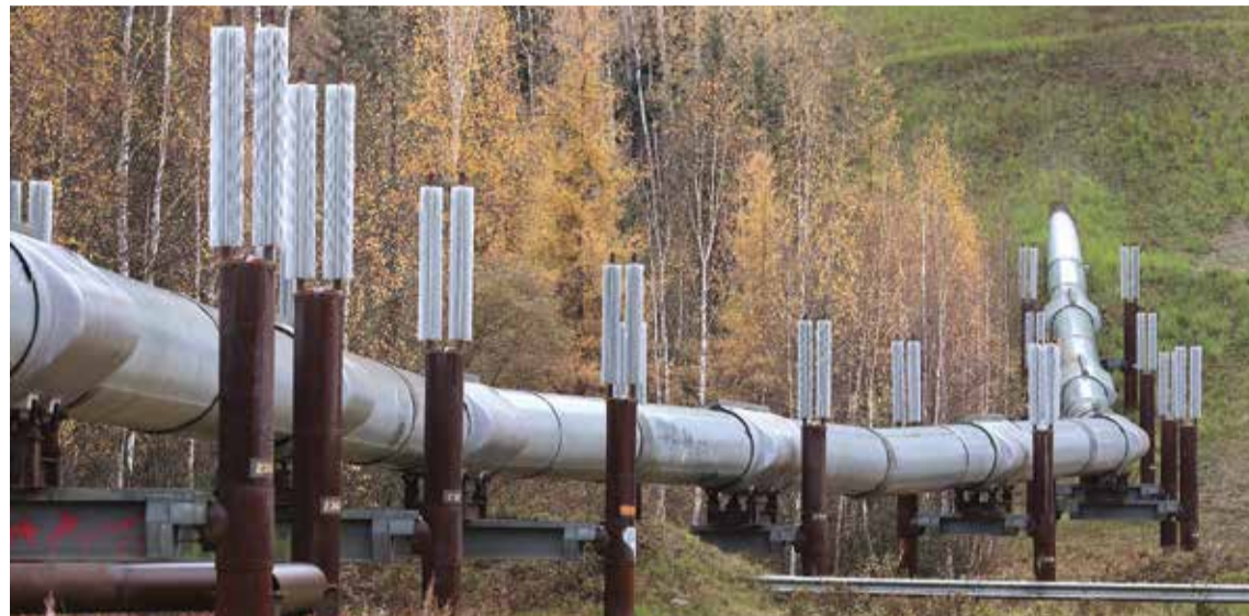
FAIRBANKS: A part of the Trans Alaska Pipeline System is seen in Fairbanks, Alaska. The 800-mile-long pipeline carries oil from Prudhoe Bay to Valdez. — AFP
