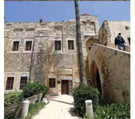
This combination of pictures shows a file picture of the 17th century Qasr al-Basha in Gaza City on April 21, 2021, where Napoleon Bonaparte slept for several nights during his campaign in Egypt and Palestine (bottom), and the same building severely damaged in Zionist bombardment.
