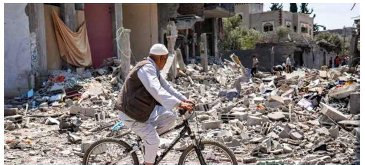
GAZA: A man rides a bicycle past the rubble of a collapsed building in the eastern side of the Maghazi camp for Palestinian refugees in the central Gaza Strip on April 15, 2024. — AFP photos
