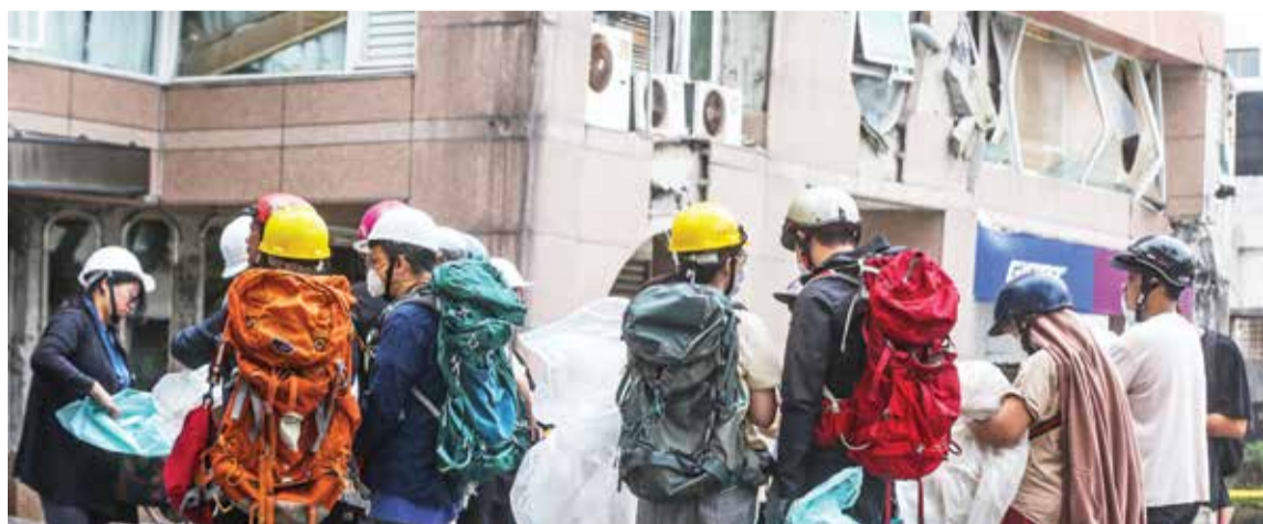
HUALIEN: Residents with safety headgear, backpacks and plastic bags prepare to salvage their belongings from the damaged Tongshuai Building following the April 3 earthquake in Hualien. — AFP
