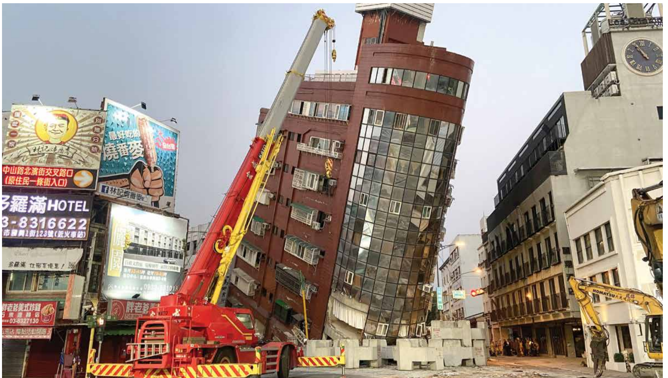
HUALIEN: This photo by Taiwan's Central News Agency shows the damaged Uranus Building in Hualien, after a major earthquake hit Taiwan's east. — AFP
