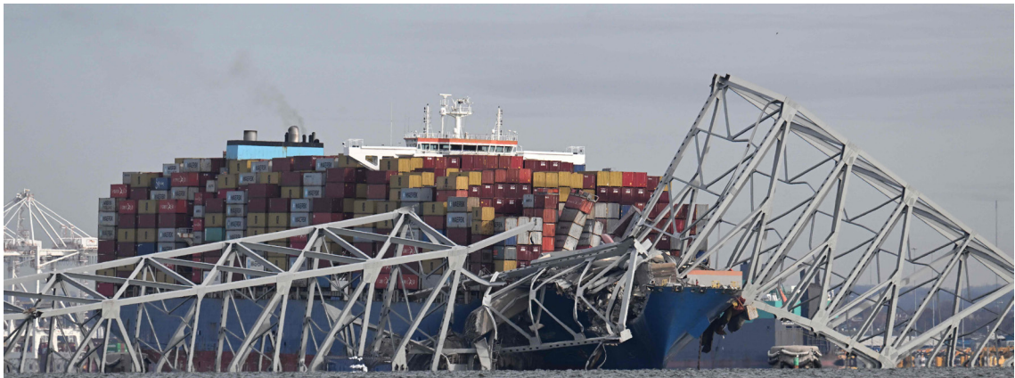
BALTIMORE: The steel frame of the Francis Scott Key Bridge sits on top of a container ship after the bridge collapsed on March 26, 2024. — AFP
