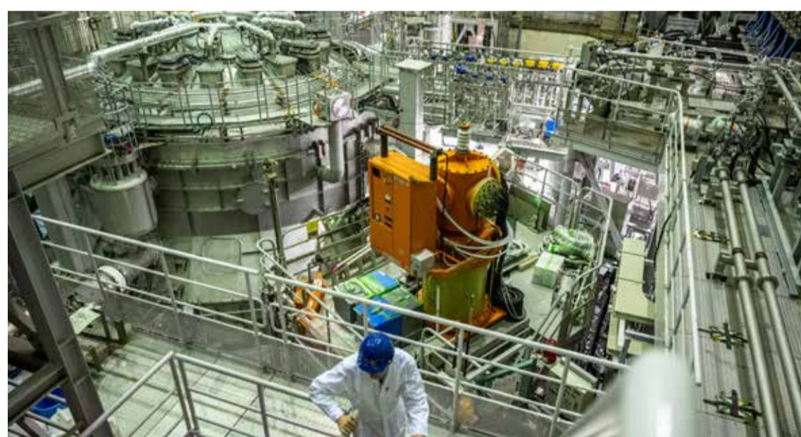
NAKA, Japan: This picture taken on Jan 22, 2024 shows a section of JT-60SA, the world's biggest experimental nuclear fusion reactor at Naka Fusion Institute in Naka city of Ibaraki Prefecture. — AFP
