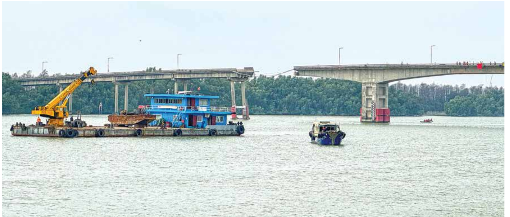
GUANGZHOU: A general view shows a section of the collapsed Lixinsha bridge over a waterway in Guangzhou, in southern China's Guangdong province on February 22, 2024. Five people were killed and three others remained missing after an empty cargo ship struck a bridge in southern China on February 22, causing part of it to collapse. - AFP
