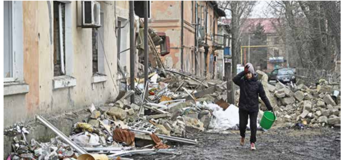
SELYDOVE: A woman walks past a residential building damaged by a missile attack in the town of Selydove, Donetsk region, on February 8, 2024. — AFP photos
