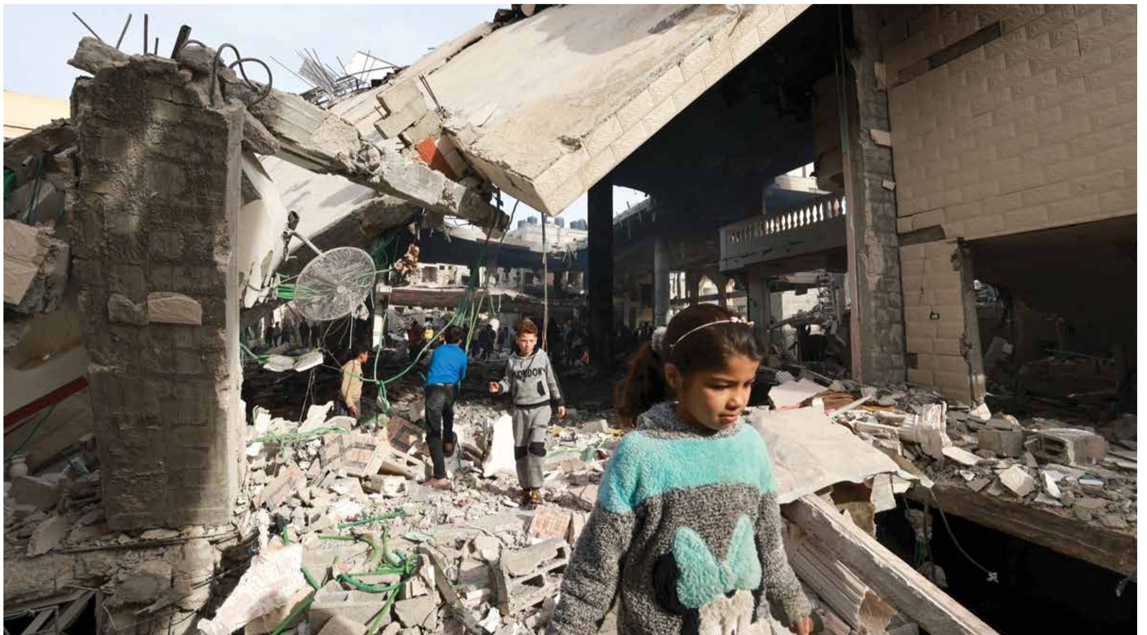
RAFAH: People inspect the damage in the rubble of a mosque following Zionist bombardment on the southern Gaza Strip on February 12, 2024. — AFP
