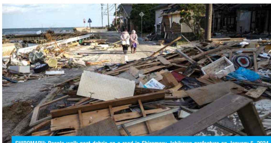
SHIROMARU: People walk past debris on a road in Shiromaru, Ishikawa prefecture on January 5, 2024, nearly a week after a major 7.5 magnitude earthquake struck the region. — AFP
