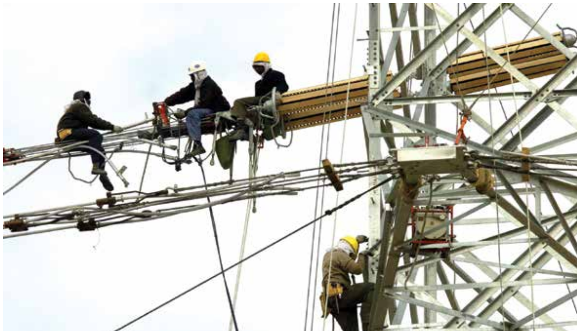
KUWAIT: (File photo) Two workers conduct a high wire job as they connect the power lines on a high voltage transmission tower on the outskirts of Kuwait City. — AFP
