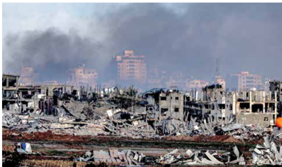
GAZA: This picture shows a view of buildings destroyed by Zionist bombardment in the central Gaza Strip from a position across the border in the Zionist entity on Jan 3, 2024. — AFP
