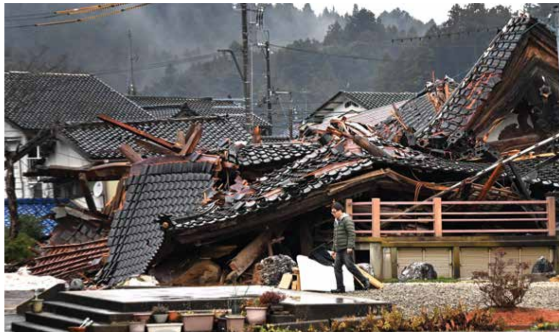
ANAMIZU: A man walks past a collapsed house in Anamizu Town, Ishikawa prefecture on Jan 3, 2024, after a major 7.5 magnitude earthquake struck the region. — AFP
