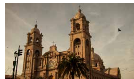
View of the Nuestra Señora del Rosario Cathedral, the main temple of the city of Tacna, in south Peru on Dec 20, 2023. The cathedral was constructed in 1875 by the French firm of Gustave Eiffel.
