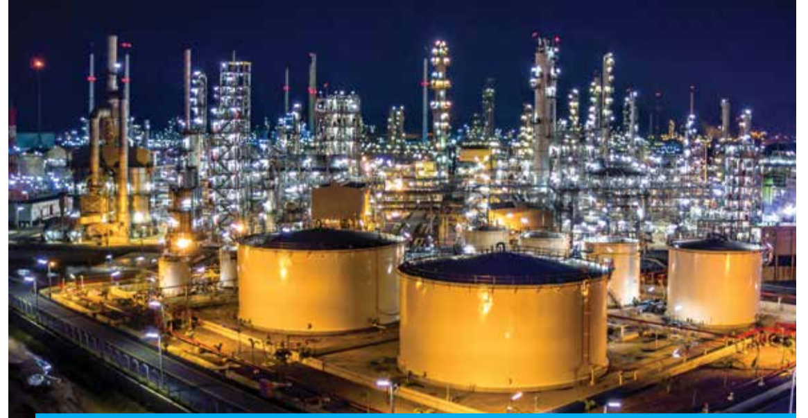
Aerial view of an oil refinery.
