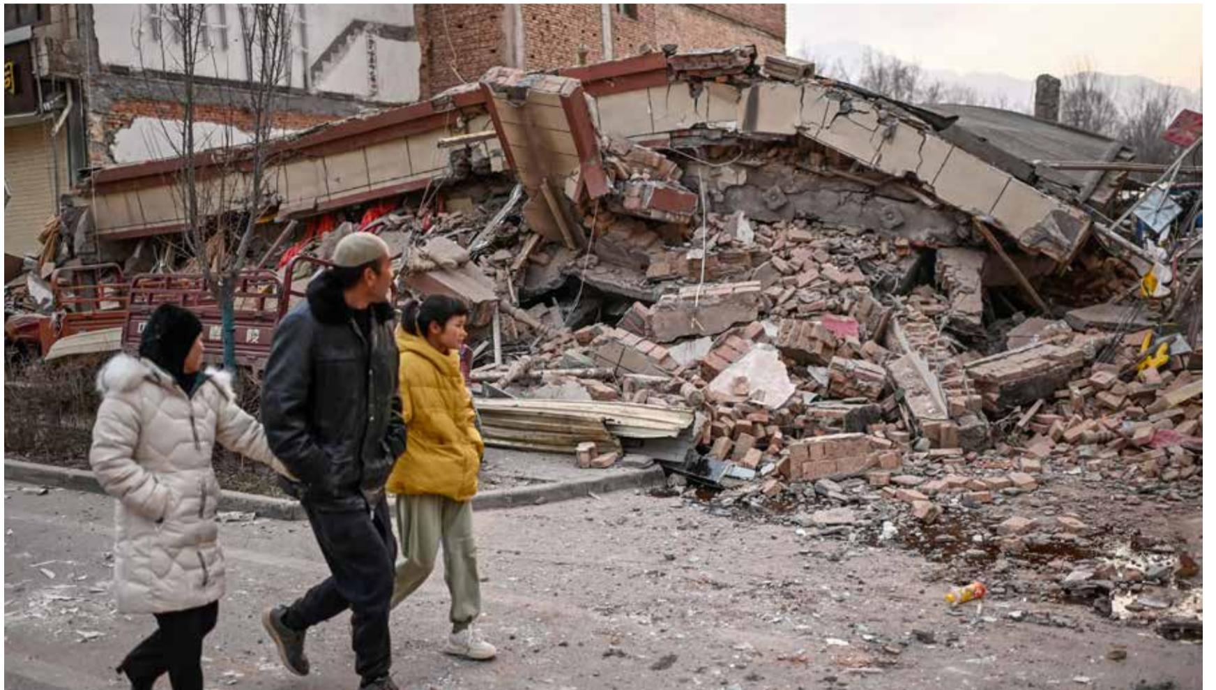
DAHEJIA: People walk past a collapsed building after an earthquake in northwest China's Gansu province on Dec 19, 2023.— AFP
