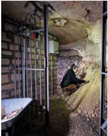
A worker sorts human bones during restoration work of Paris' Catacombs.
