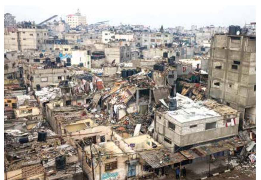
RAFAH, Palestinian Territories: This picture shows the damages following Zionist entity bombardment in Rafah in the southern Gaza Strip on December 13, 2023. — AFP
