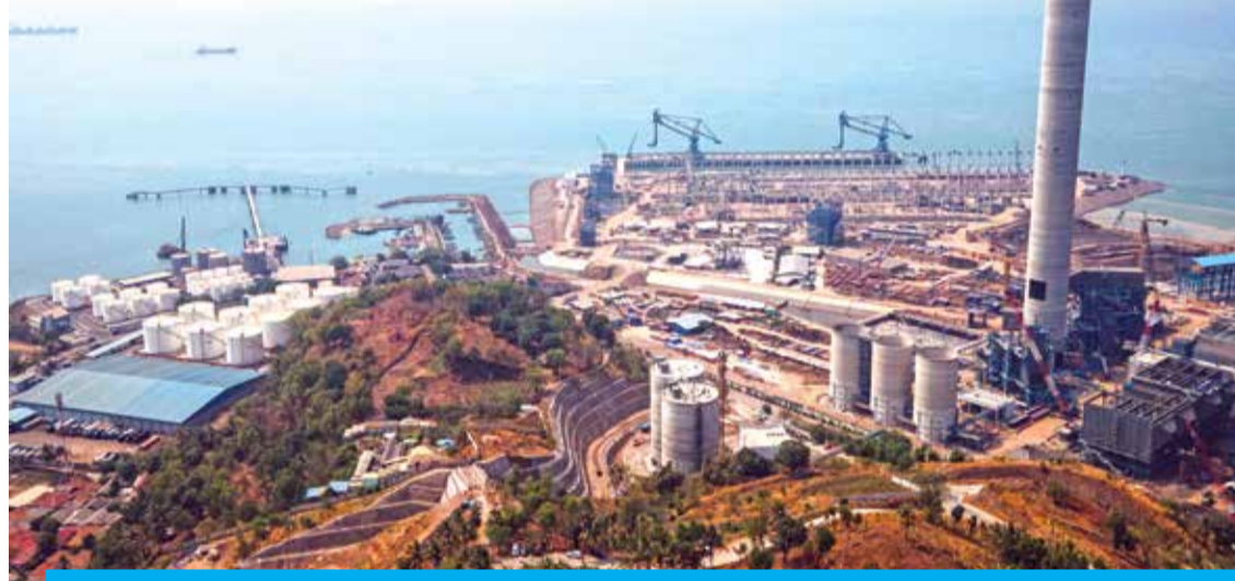
CILEGON, Indonesia: This picture taken on October 31, 2023 shows new construction at the Suralaya coal-fired power plant in Cilegon, Indonesia's Banten province. As countries gather in Dubai for crunch climate talks, the future of polluting fossil fuel coal will be high on the agenda. -- AFP
